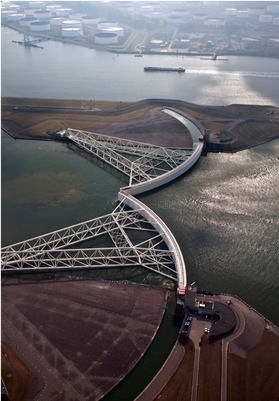
A movable storm-surge barrier in Rotterdam, Netherlands, in its closed position
